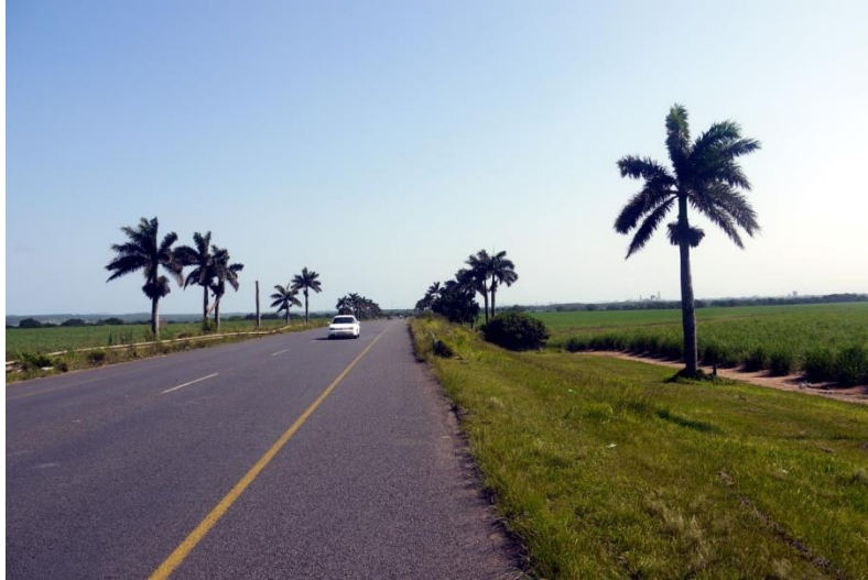
Plate 11 The P106 near Esikhawini looking towards the proposed site.
